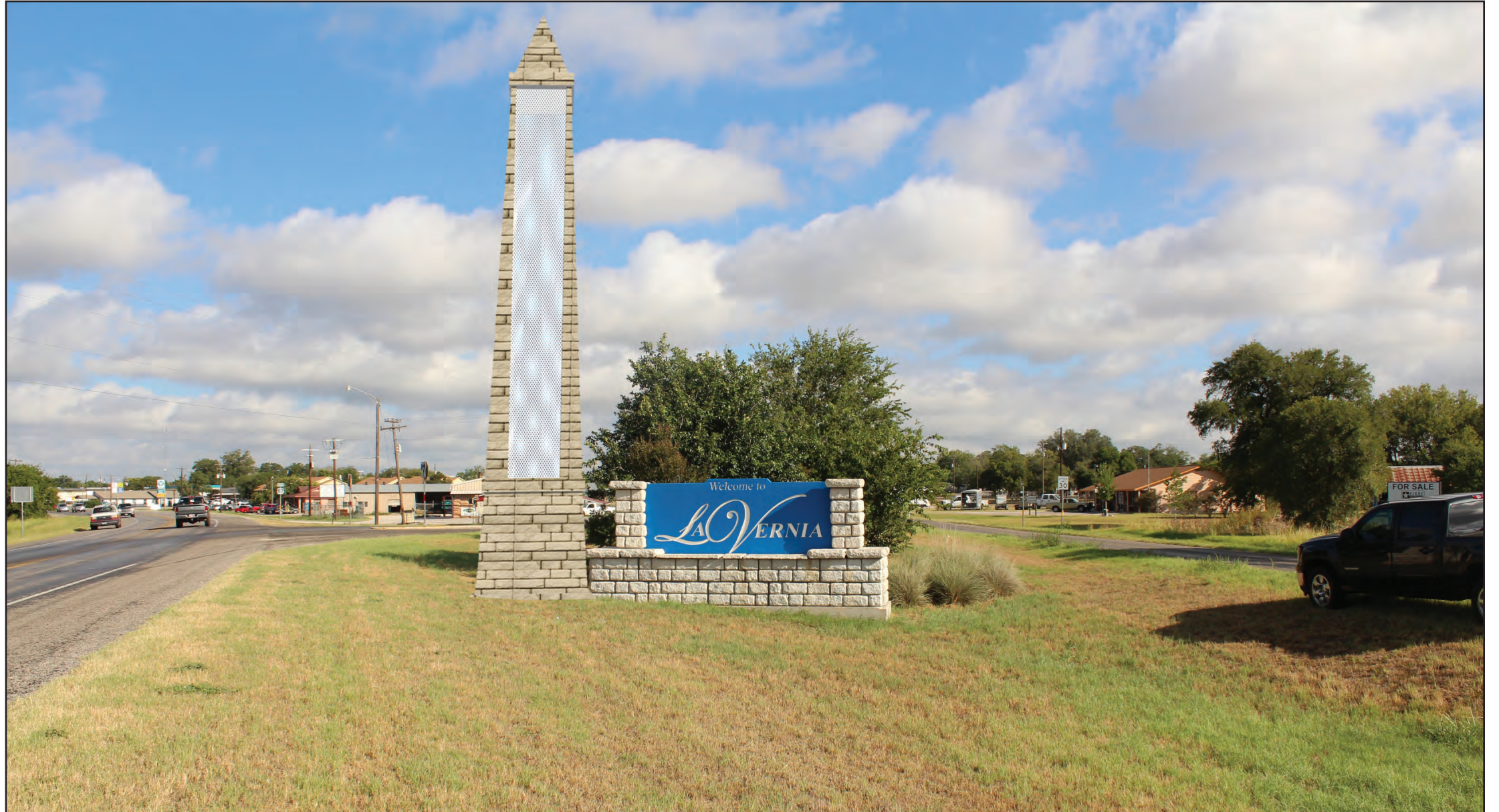
Figure 45: Proposed Gateway Installation on Highway 87 south of La Vernia
