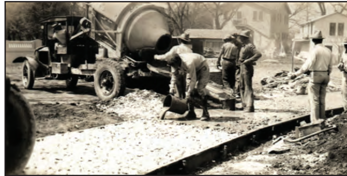
Figure 12: Sidewalk Construction along Texas Highway 66 in Pleasanton, 1935 Source: Texas Transportation Museum - Hemphill
